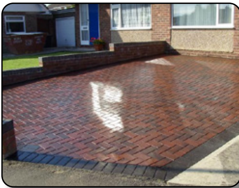
Concrete cures and sealers
